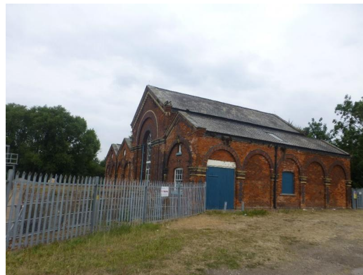
Plate 27: View of Dirtness Pumping Station looking north-east
