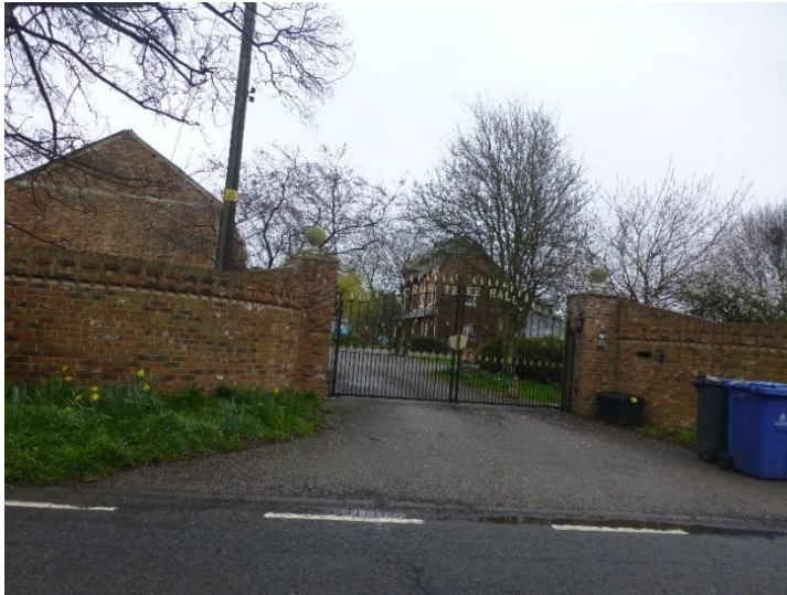
Plate 4142: View of Crow Tree Hall looking east
